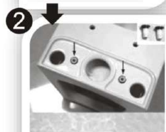
Attach cistern bolts into pan Tighten bolts from underneath
